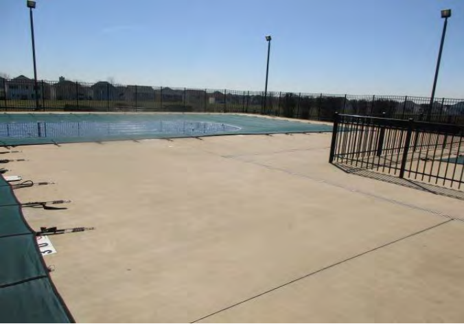
Overview of concrete pool deck
