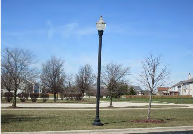
Light pole and fixture at parking lot
