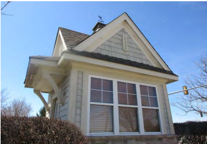
Windows at guardhouse building
