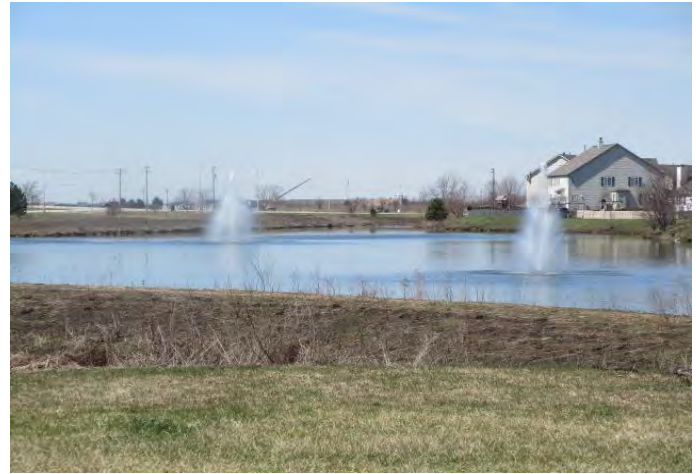
Pond aerators are replaced operationally
