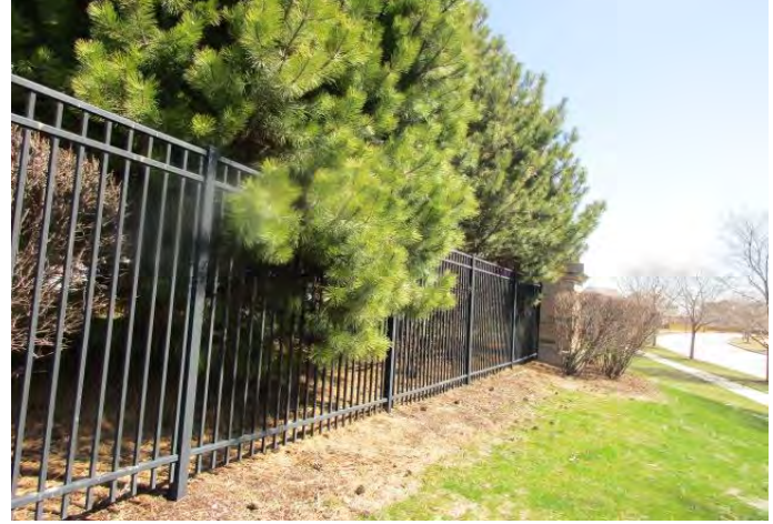
Aluminum picket fence near main property entrance
