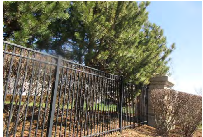
Aluminum picket fence near entrance monument wall
