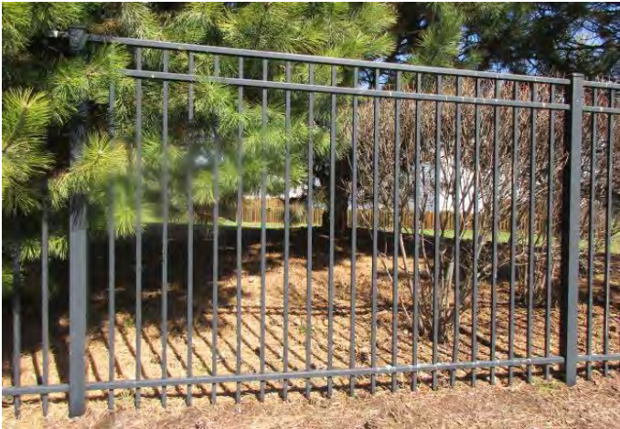
Aluminum picket fence near entrance monument wall
