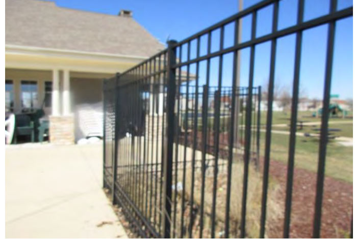
Overview of aluminum fence at perimeter of pool
