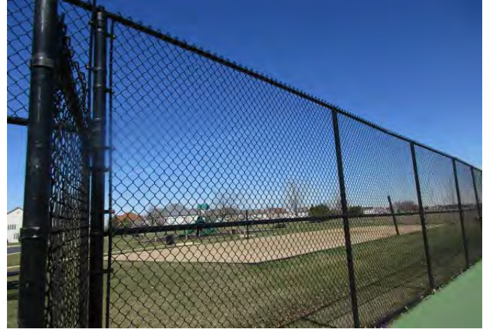
Chain link fence at tennis court perimeter
