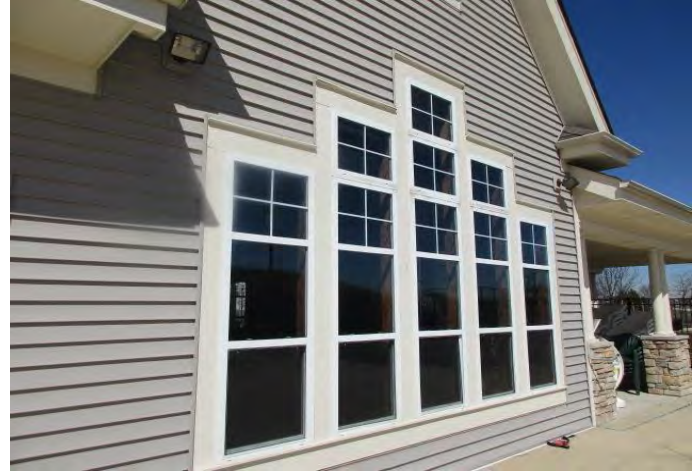
Pool-facing windows at clubhouse
