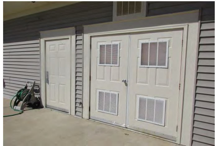
Exterior doors at restroom & pool equipment room
