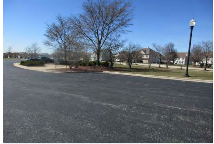
Asphalt pavement at parking lot at clubhouse
