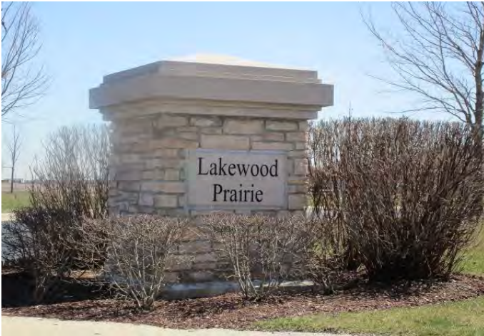
Masonry signage pier at clubhouse parking lot
