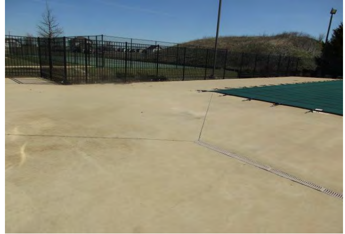
Overview of concrete pool deck
