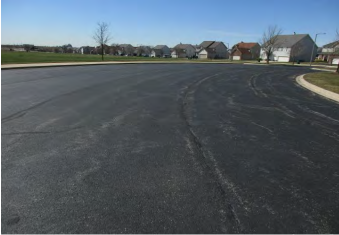
Asphalt pavement at parking lot at clubhouse
