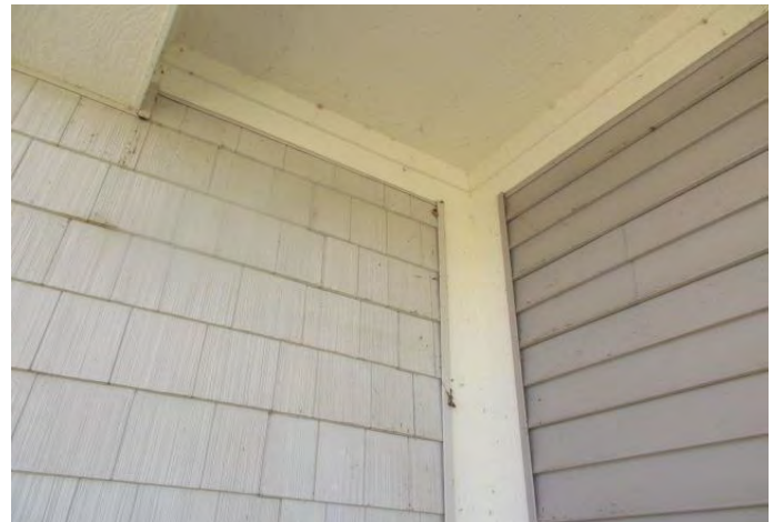
Vinyl siding with hardboard trim at clubhouse
