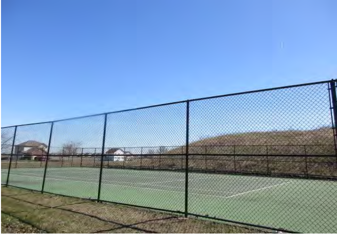
Chain link fence at tennis court perimeter
