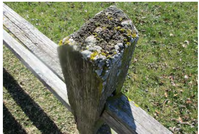
Wood deterioration at top of fence post
