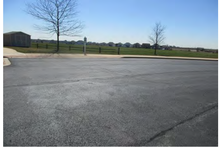
Asphalt pavement at parking lot at clubhouse
