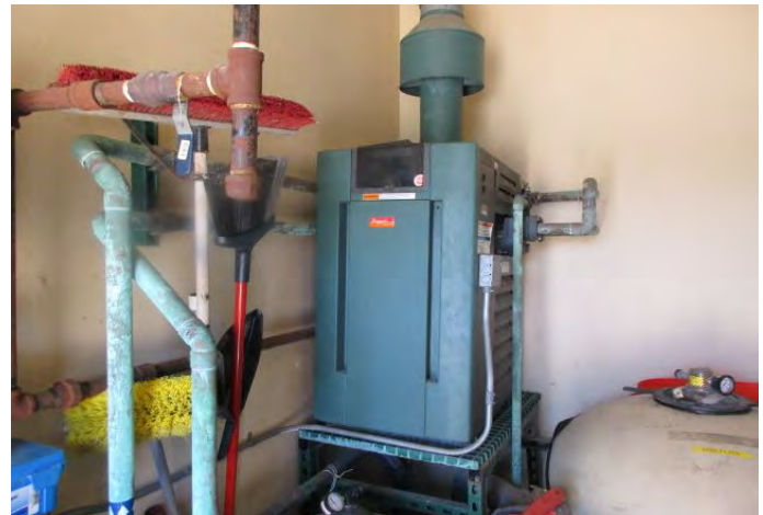
Heater for wading pool
