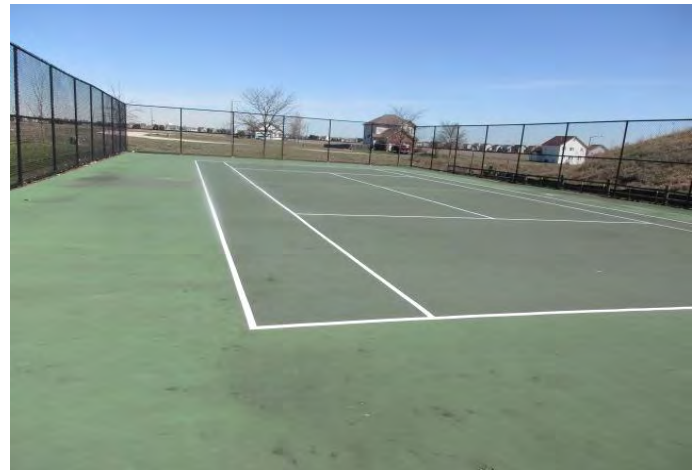
Typical condition at tennis court pavement
