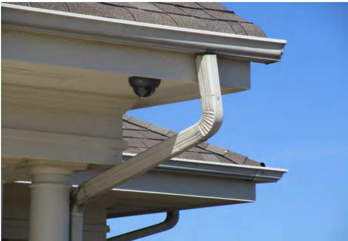
Gutters and downspouts at roof eaves
