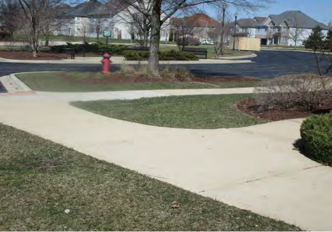
Concrete sidewalks at clubhouse
