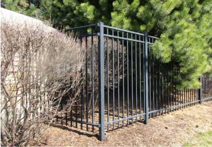
Aluminum picket fence near main property entrance
