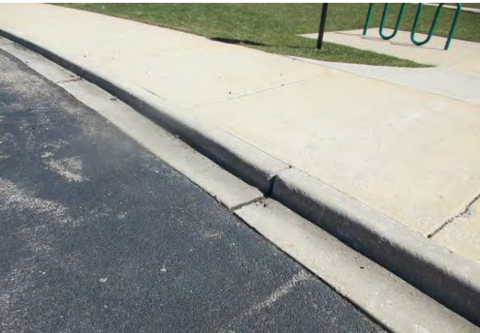
Raised curb and gutter at perimeter of parking lot
