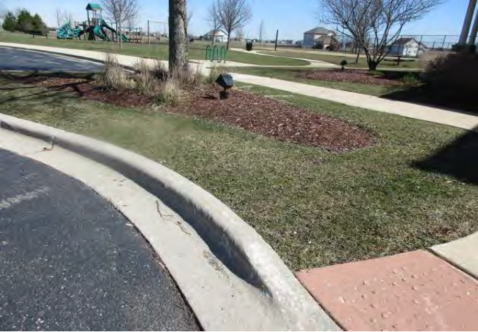
Concrete curb at handicap entry ramp
