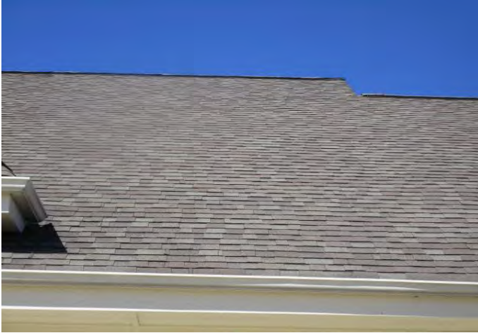
Overview of asphalt shingle roof at clubhouse
