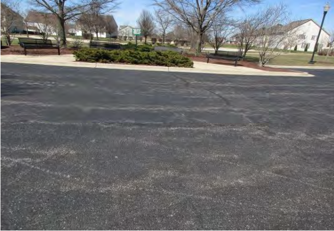
Asphalt pavement at parking lot at clubhouse
