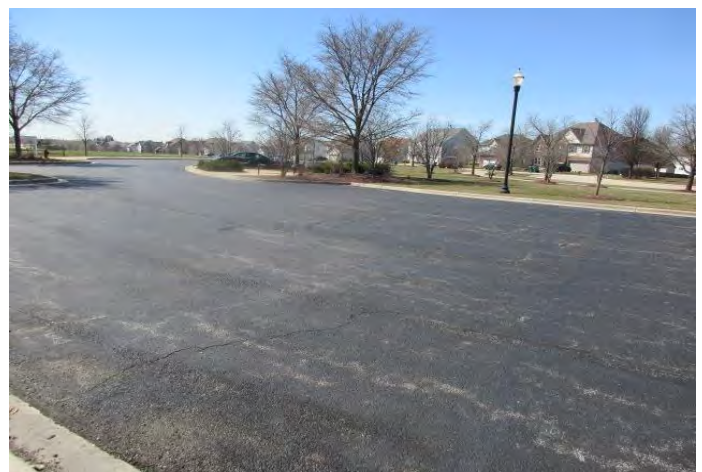
Pavement is in fair overall condition
