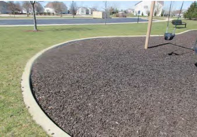
Rubber resilient ground cover at playground area
