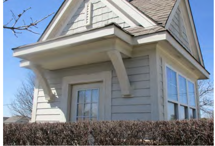
Overview of guardhouse building
