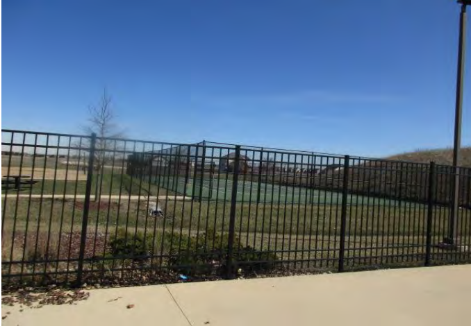
Overview of aluminum fence at perimeter of pool
