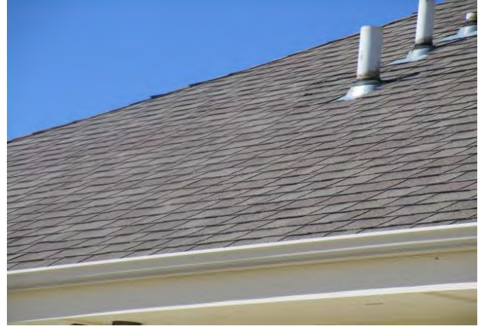
Overview of asphalt shingle roof at clubhouse
