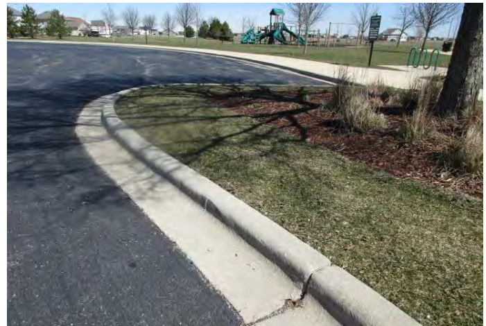
Raised curb and gutter at perimeter of parking lot
