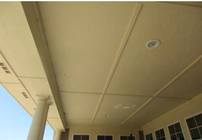
Soffit at covered patio area at clubhouse
