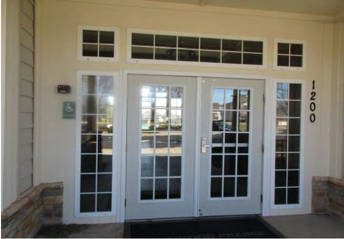
Entry doors and surrounding windows at clubhouse
